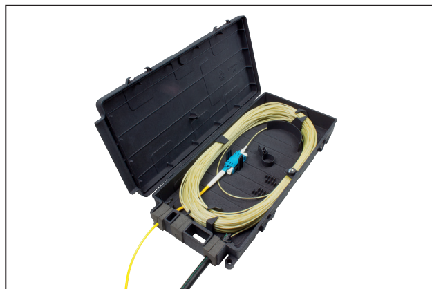
Customer Connection Enclosure
