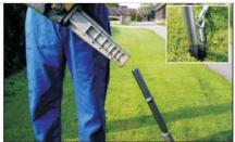
7. Caution! Two man lift. Lift the breaker onto the shank and continue driving the anchor until the protective sleeving just reaches ground level. This will leave the top eye approximately 150mm above ground level. Driving the anchor past this point can make loadlocking difficult.
