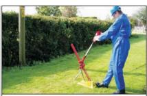
11. The anchor will rotate through the ground into its loadlocked or working position. This will normally take an anchor bodies length (approximately 250mm). Once the anchor has reached its working position the load will be felt on the jack.
