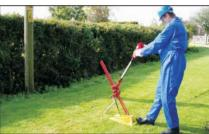
11. The anchor will rotate through the ground into its loadlocked or working position. This will normally take an anchor bodies length (approximately 250mm). Once the anchor has reached its working position the load will be felt on the jack.
