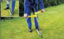
8. Caution! Two man lift. Remove the breaker from the shank and using the rod removers, withdraw the drive rods from the ground. Caution! Rods and couplers may be very hot. Wear gloves. In reasonable ground the installation process should not take more than 3-4 minutes. In very hard ground up to 10 minutes may be needed.
