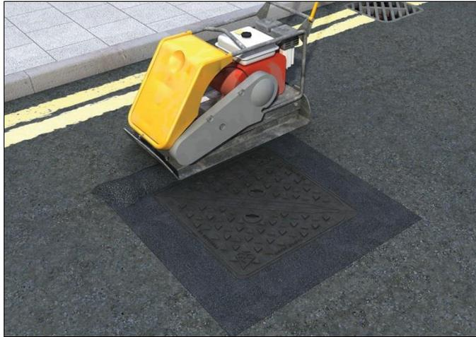
11.14 An Ultracrete Envirobond HA104, Ultracrete Envirobond HA104 Flowable or Ultracrete M60 and Ultracrete M60F installation should not be trafficked for a minimum of two hours following completion of the installation. This may be reduced to one hour for an Ultracrete PY4 installation.
