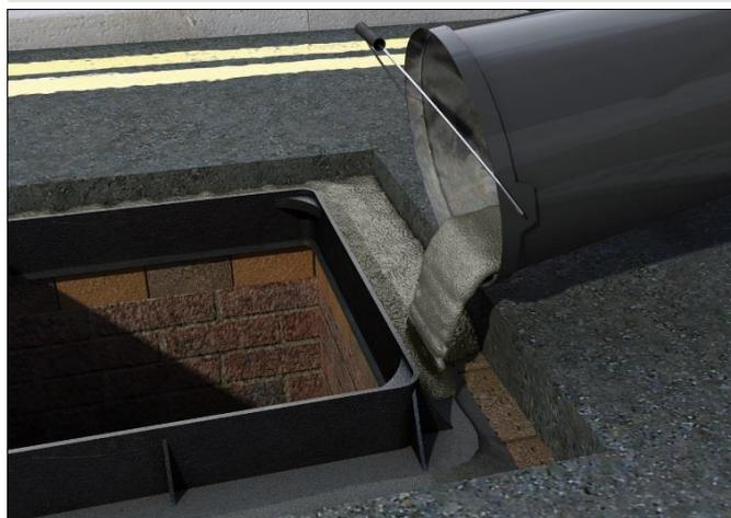
11.11 Once Ultracrete QC10 and Ultracrete QC10F has reached initial set, all vertical edges of the excavated area and the manhole frame are sprayed with Ultracrete Seal and Tack, ensuring all surfaces are covered (see Figure 6).
