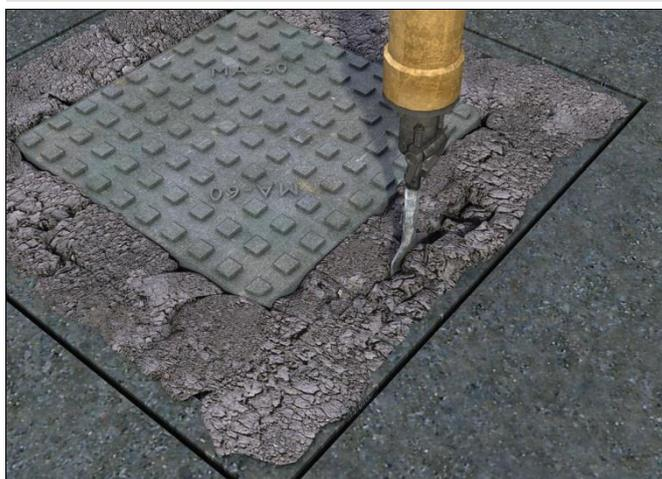
10.4 All old bedding mortar is removed and the supporting structure cut back or loose bricks removed until a sound base is achieved.
