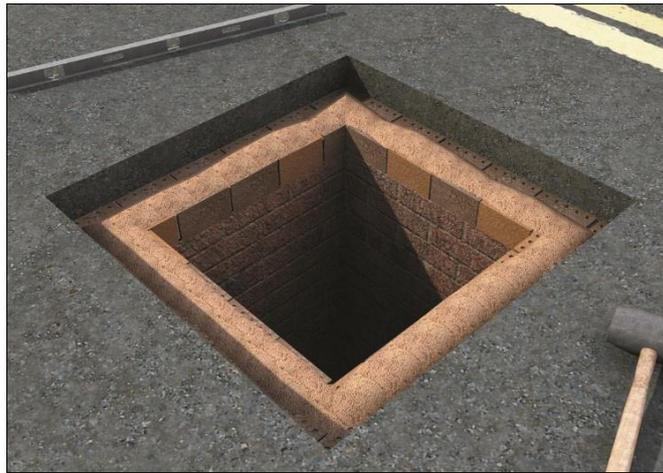
11.2 When packing materials are used to support and level the frame, they must be compatible with the bedding mortar to be used. The Certificate holder can advise on suitable materials.
