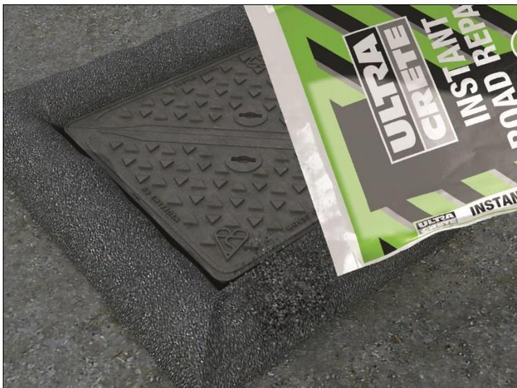
Figure 8 Final compaction of Ultracrete Instant Road Repair
