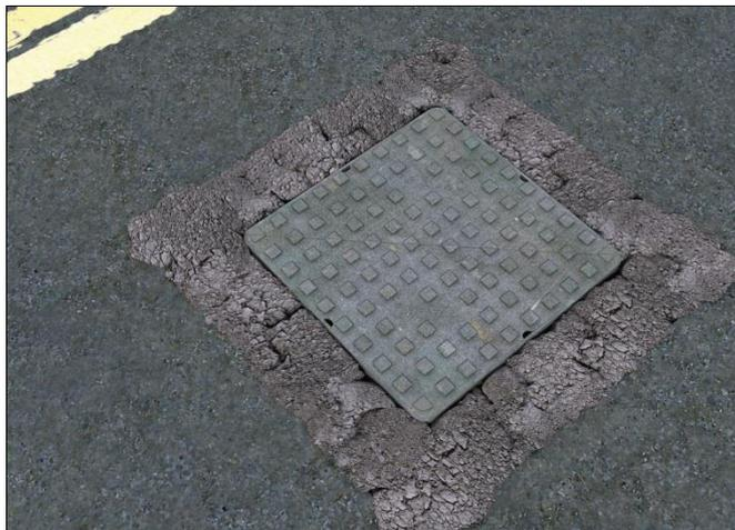
10.2 The supporting structure must be of adequate size and strength to support the frame, cover and expected loading.
