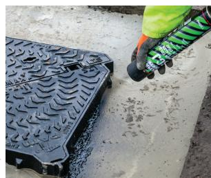
A cold joint sealer that is applied onto vertical edges and surface base before the application of asphalt.
