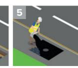
A temporary deferred set is then applied to the surface until such time the hot lav asphalt arrives. (subject to material availability).
