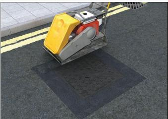
11.14 An Ultracrete Envirobed HA104, Ultracrete Envirobed HA104 Flowable or Ultracrete M60 and Ultracrete M60F installation should not be trafficked for a minimum of two hours following completion of the installation. This may be reduced to one hour for an Ultracrete PY4 installation.
