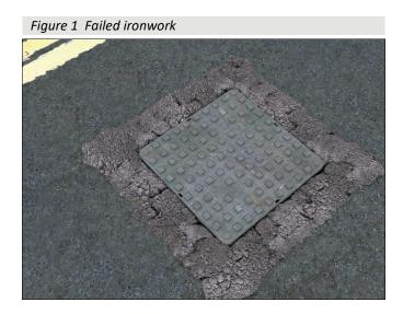
10.2 The supporting structure must be of adequate size and strength to support the frame, cover and expected loading.
