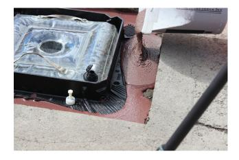
The inflatable device that acts as a dam allowing a flowable mortar installation around an access frame within seconds.
