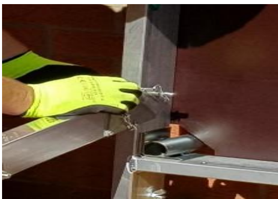
3. Attach each main leg to the underside of the Platform, Look for "Normal Use" sticker. Red sticker right hand side and green sticker left. Always fit pins so the R clip on the underside of the Platform.
