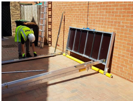
1. Lay out the components ready for assembly with the Platform/Dec against the wall with wheels or Rolling Window bar on the ground as shown.
