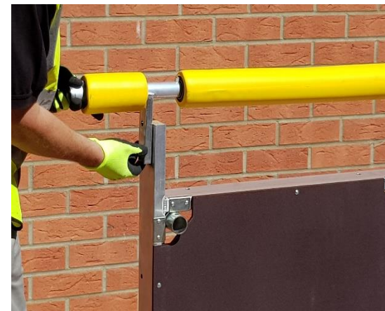
2. Attach the Dec wheels or the 2.4metre Rolling window bar (optional extra). We have used the Rolling window bar for this erection sequence.
