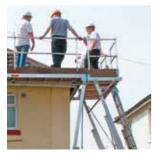
**Corner Kit:** Allows access to large box-end gutters or can provide a continuous working platform around corners.
