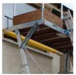
**Rolling Window Bar:** Allows an Easi-Dec to be positioned across a window or fragile wall surface with an even distribution of weight.
