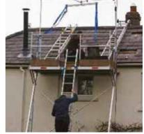
Solar Platform has been specifically designed to allow safe access up to roof level for solar installation, repair and maintenance. The Solar Platform is a 2m wide platform on adjustable legs with a rolling window bar, strap operated legs and a purpose designed hoist for lifting Solar Panels to roof level.
