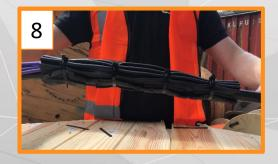
Over tightening of the cable ties can risk damaging the tubes inside. they can be unfastened, if required, using the release button on the head. Remove tails from the cable ties using snips
