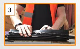
Wrap the EM-Wrap round the tube bundle and drops with the four tabs on the outside.
