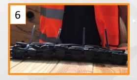
Check that the wrap does not move over the bundle and tighten cable ties where necessary.
