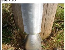
Protect the cable going up the pole with the steel or plastic capping.
