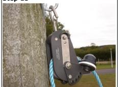
Feed the pulling bond through the pulley at the cable dispenser pole.
