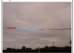
Continue to pull the cable across the span until there is enough cable left on the drum to locate the preconnectorised end into the CBT Terminal Block.
