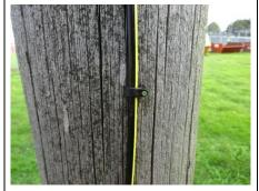
Secure the feeder cable down the pole using pole cleats.
