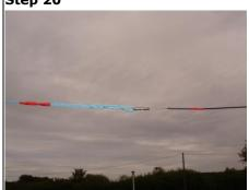
Pull the pulling bond and cable across the span. Care should be taken to ensure that there is no risk to third parties
