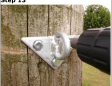
Attach the Mounting Clamp to the pole at the correct position.
