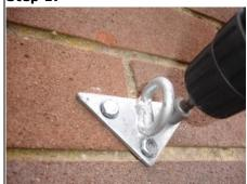
Attach the Mounting Clamp to the house at the correct position.
