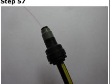
Fit the connector to Drop Cable.
