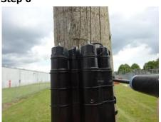
Re-attach the connector housing to the base. The housing is designed for either top or bottom entry of the drop cables.
