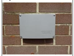
At the building end fit the CBT External Customer Termination Box in a suitable position. This could be inside or outside the building.
