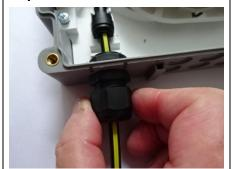
Tighten gland sealing nut.
