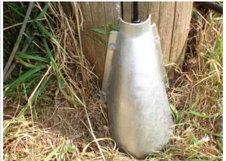
Fit the capping adaptor to the base of the pole.
