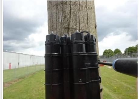
Re-attach the connector housing to the base. The housing is designed for either top or bottom entry of the drop cables.
