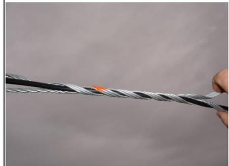
Pull the cable to the required tension and fit the helical tension clamp at the pole/house.
