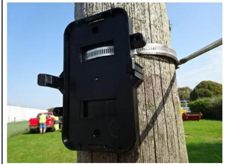
Attach the base to the pole using the steel banding provided. Alternatively, the base can be attached to the pole using wood screws.
