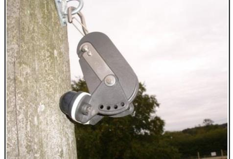
Attach a suitable pulley to the Mounting Clamp.
