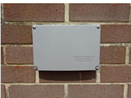
At the building end fit the CBT External Customer Termination Box in a suitable position. This could be inside or outside the building.
