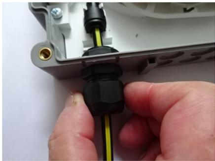
Tighten gland sealing nut.
