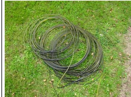
Remove and fleet sufficient cable from the drum to enable the cable can be installed into the u/g joint.
