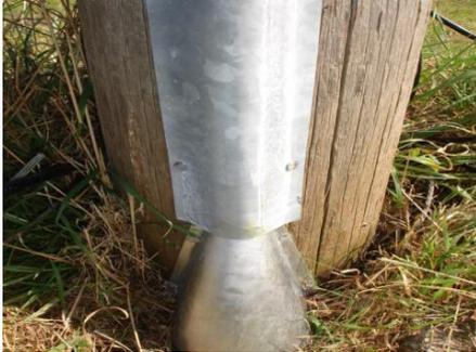
Protect the cable going up the pole with the steel or plastic capping.
