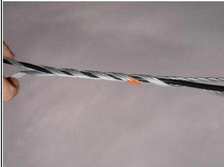
Fit the helical tension clamp to the cable and mounting clamp at the cable dispenser pole.
