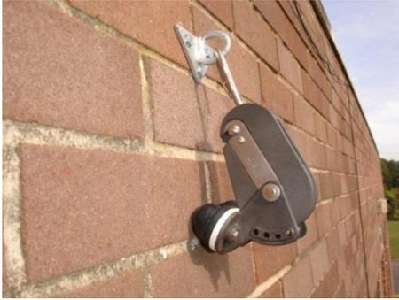
Attach a suitable pulley to the Mounting Clamp.
