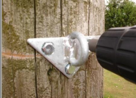
Attach the Mounting Clamp to the pole at the correct position.
