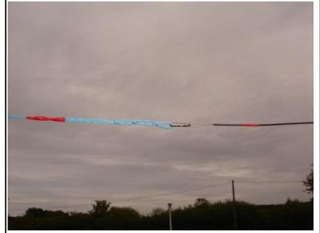
Pull the pulling bond and cable across the span.
