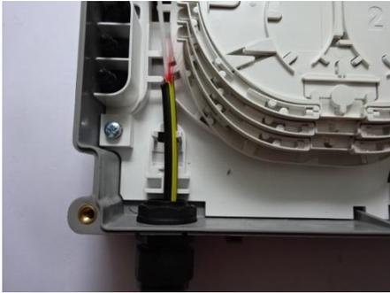
Insert the drop cable through gland and position approximately 65mm from the lowest face of the box.
