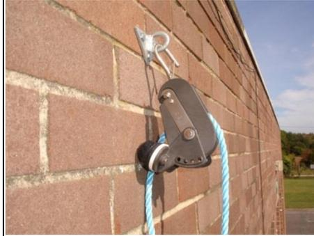
Pass the pulling bond through the pulley at the remote pole/house.
