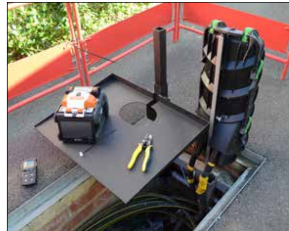
Pitmate Mobra Arm Bracket (S83-7626) mounted with Splicer's Worktray (S83-7629)
