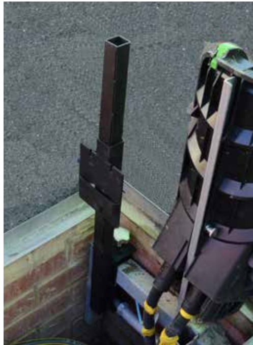
Pitmate Mobra Arm Bracket (S83-7626) fitted to Mobra frame
