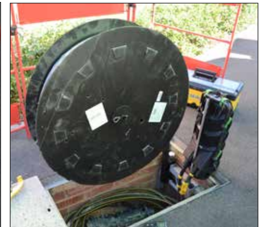
Pitmate Mobra Arm Bracket (S83-7626) mounted with CBT Arm System (S83-7624)
