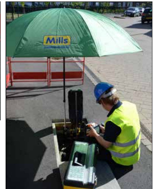
Pitmate Umbrella Clamp (S83-7625) mounted on to Mobra frame
